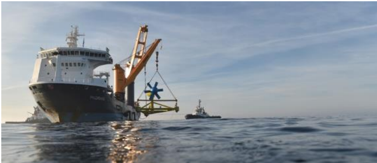
Deployment of the Sabella D10 turbine
